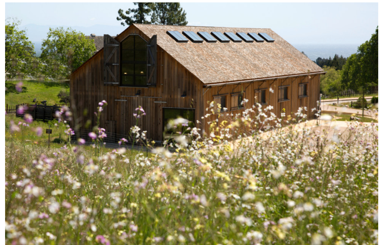
▲ Renovated Hay Barn
