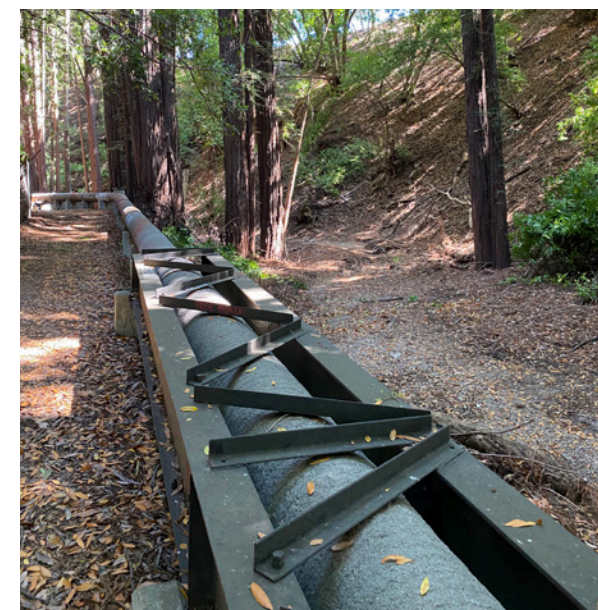
▲ Jordan Gulch above grade sewer
