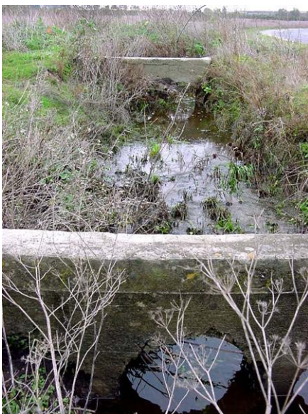
Fig. B.6 Concrete headwalls in drainage
