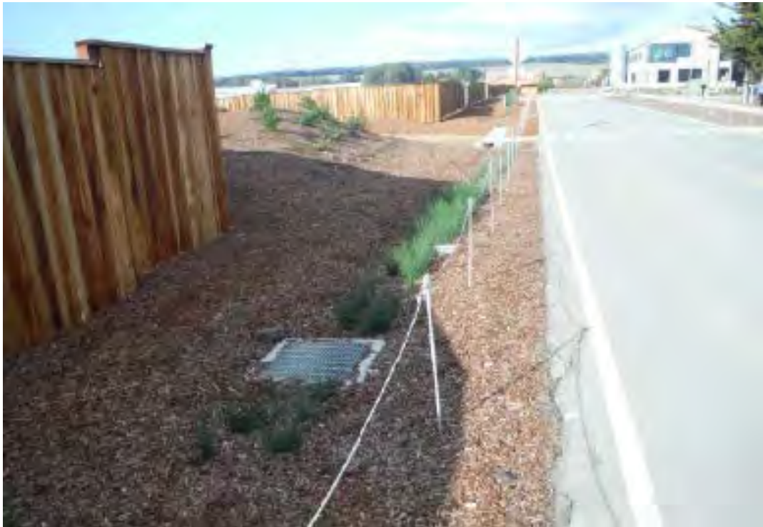
Photo #1: NOAA Outfall east side drop inlet, post-construction. November 2017.
