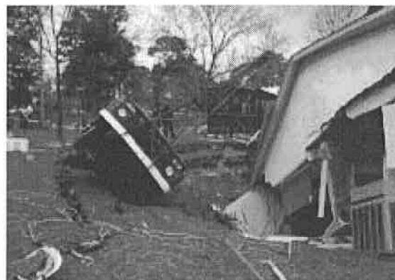
Fig. 29. Water well drilling near this Florida home triggered a sinkhole collapse beneath both the drill rig and the house.
