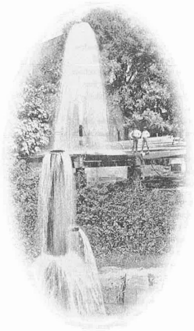
Fig. 51. Water flowed abundantly and forcefully from the first wells drilled into Texas' Edwards Aquifer in 1897. Now, with large water withdrawals from the aquifer, water discharge is restricted.
