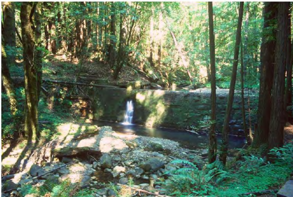
Figure 6-5. Laguna Creek Diversion Dam
