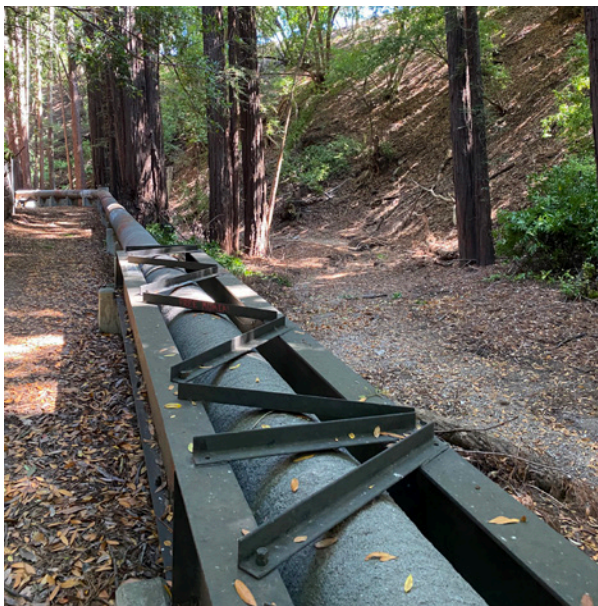
▲ Jordan Gulch above grade sewer
